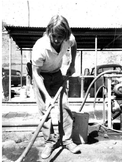
Don at Mogo Creek NSW working for Hodge Industrial – installing underground petrol tanks and bowsers for petrol stations.
